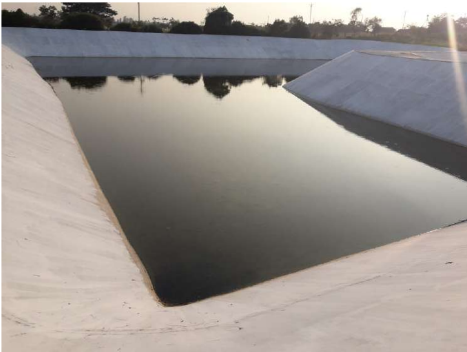
15 Days Storage Tank-2
