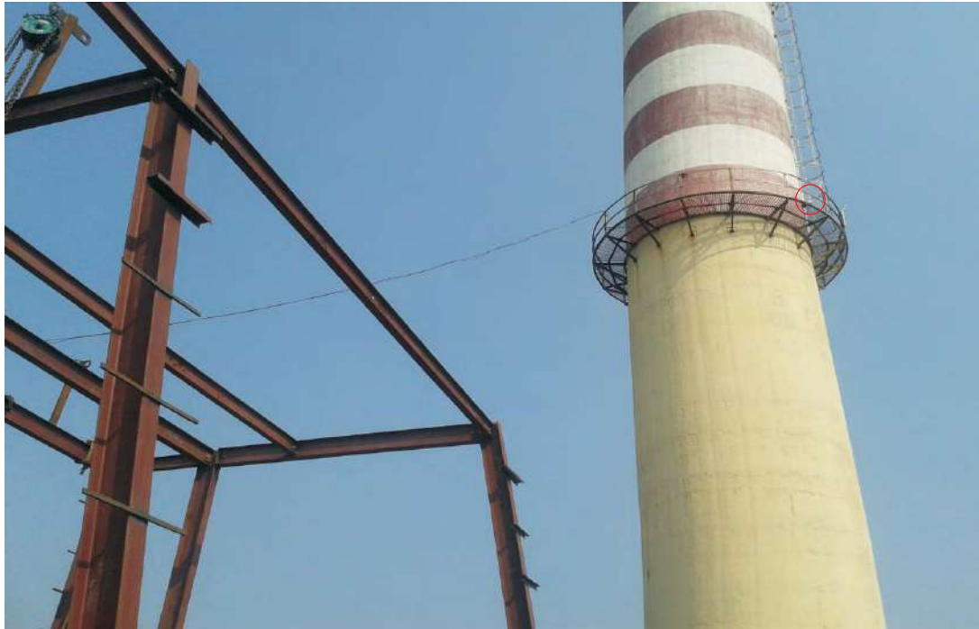
Dust monitor unit for Total Particulate Matter for 75 mtr.height stack
