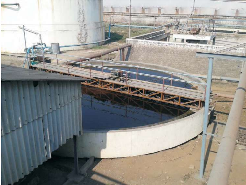
Secondary clarifier old stream
