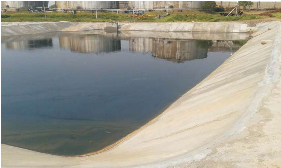
R.C.C. with Geomembrane paper lining laid for Lagoon No.1
