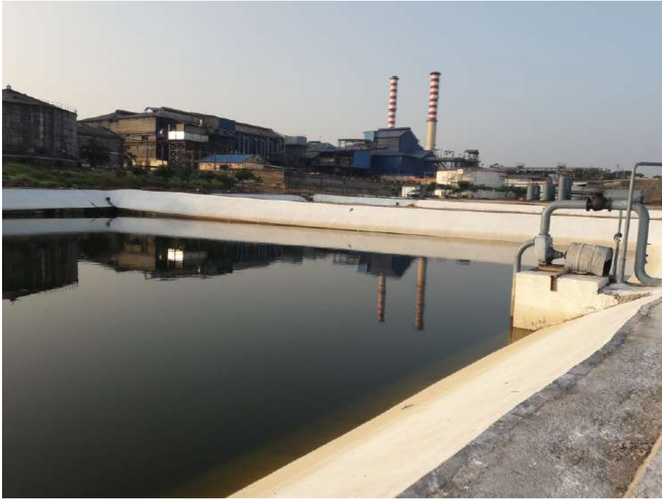
15 Days Storage Tank-1
